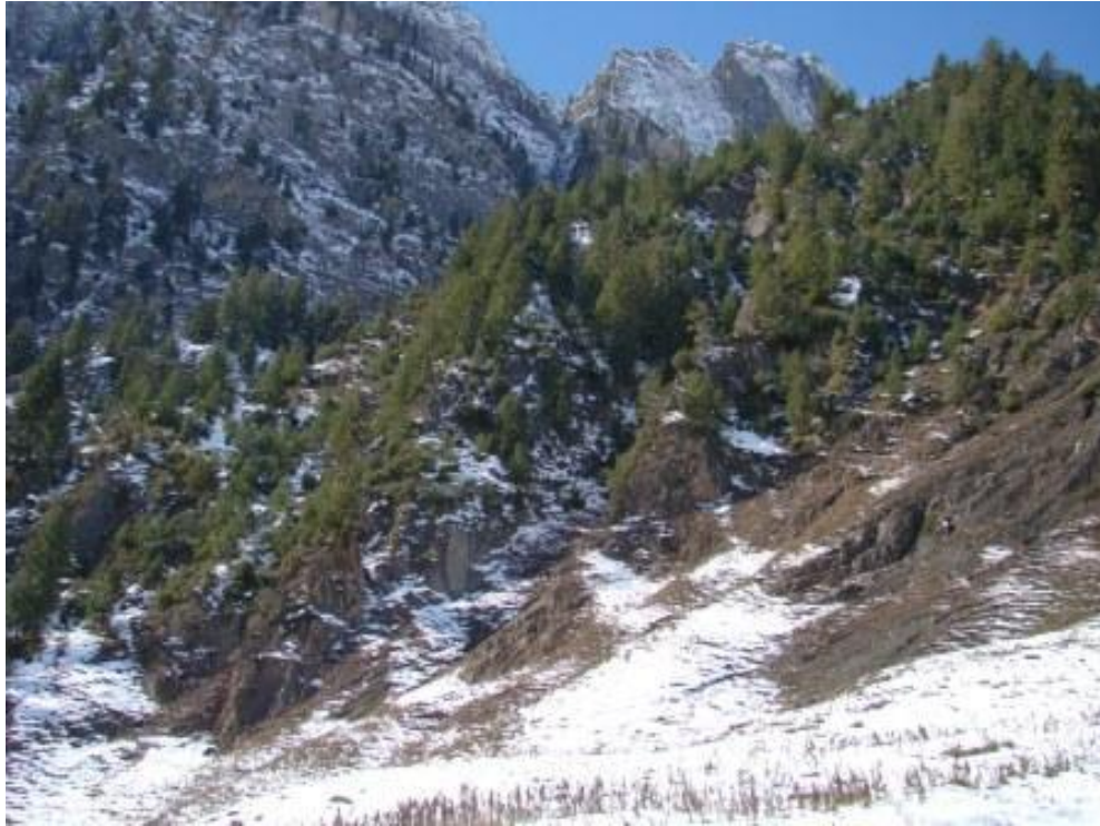
Fig 37 A View of Shear Zone near toll barrier Sonamarg
