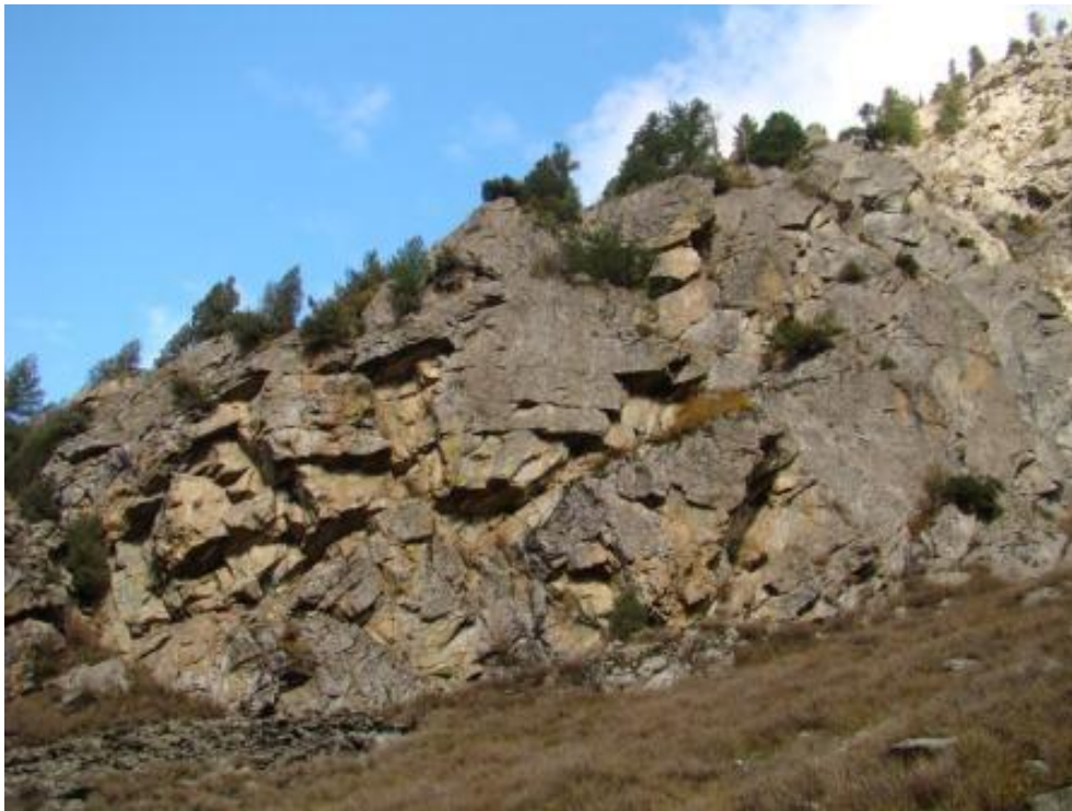
Fig. 28 A View of joint sets near West portal area
