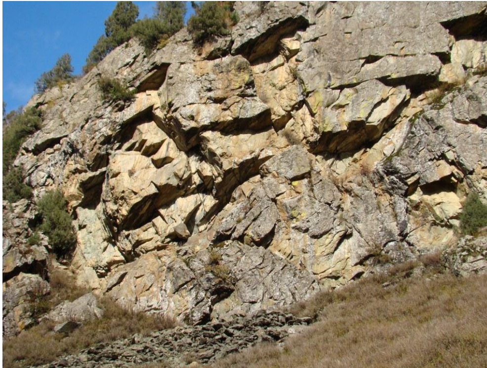
Fig.30 A View of Open joints set
